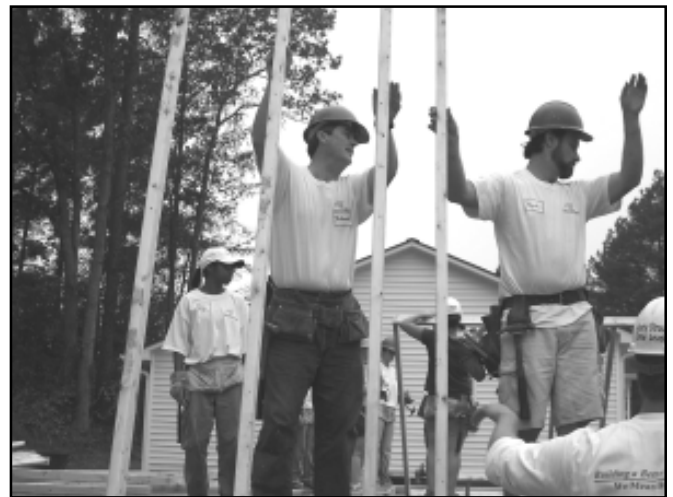
Robert W. Jones and fellow SunTrust employees raise a wall.
