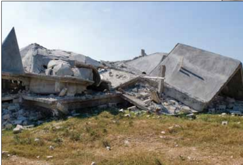
Above: Homes and buildings just blocks from the Habitat neighborhood in Cabaret were destroyed. Of 183 Habitat homes in the area, initial reports indicate that only eight sustained damage; by comparison, it is estimated that 8,000 non-Habitat homes were destroyed in the surrounding areas.
